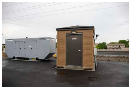
Top: Interior of control building. Bottom: Prefabricated control building & generator. Left: Installation of reinforced polymer wet well.
