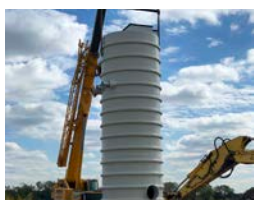
FRP Lift Station Eases Problematic Roadblock, to Provide Decades of Durability Page 2
