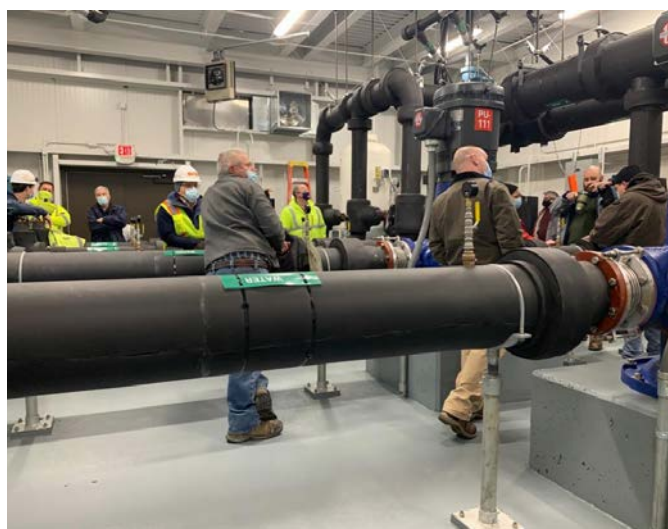
Top: Completed upgraded potable water pump station at W. Averell Harriman State Office Building Campus.
