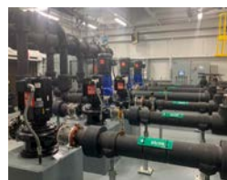
Potable Water Pump Upgrade Continues to Push Through Unforeseen Setbacks
