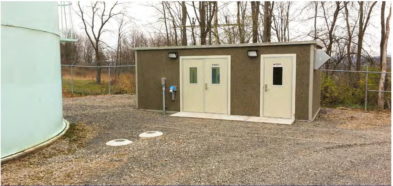
*Above: The exterior of one of three housed booster systems, delivered and installed in Preston County, W. Va. Durable, prefabricated concrete structures were chosen for this project and shipped complete to the job site.*
