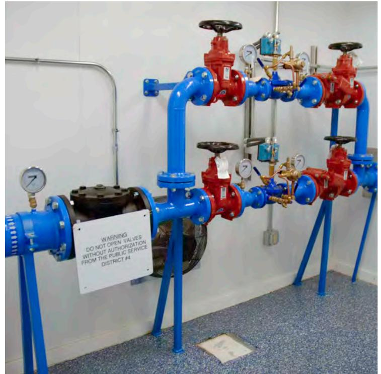
*Above: Interior of one of three booster systems delivered to West Virginia. Right: Interior of one of three pressure reducing valves (PRV) stations delivered to West Virginia. Below: Chemical room of housed booster stations.*
