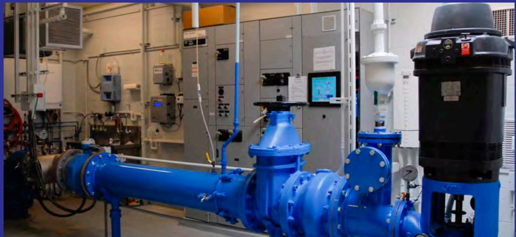
*A 12 inch ultraviolet treatment unit was added to existing well piping and is housed within the Village of Romeoville's Lake Strini well-house.*
