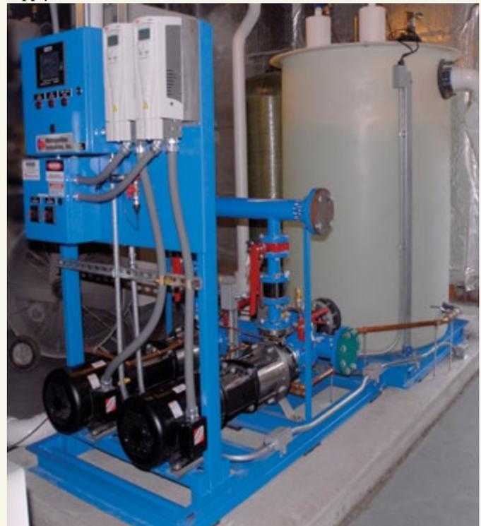
*Combination pump system and break tank system with a protected water supply designed with a flow rate of 120 gpm.*
