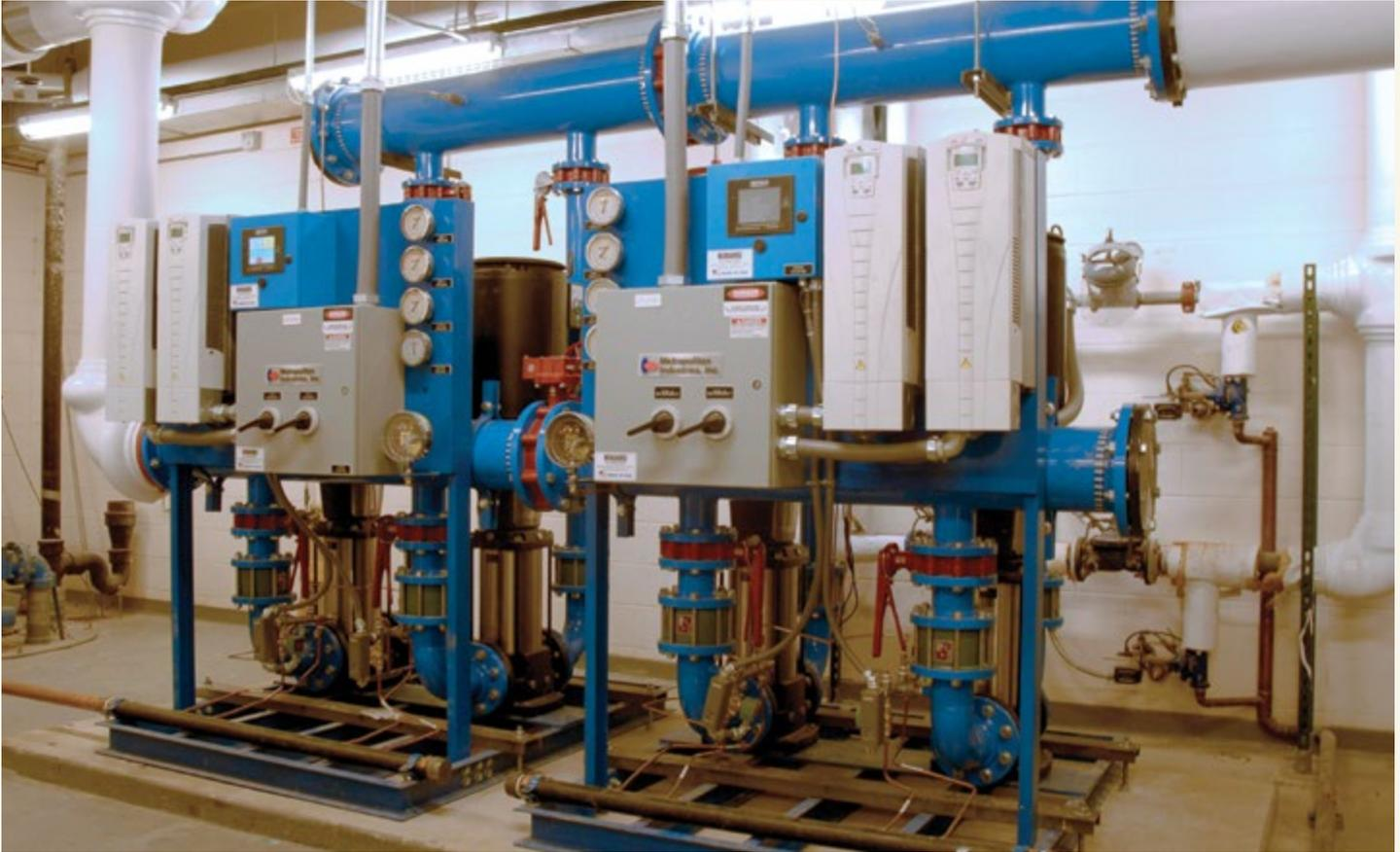
*New booster pump system designed with potential future expansion in mind.*
