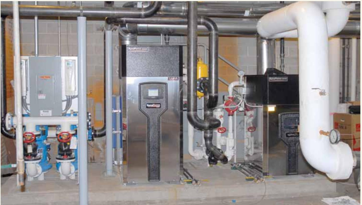
Pictured are the new hybrid boiler system package and the primary pump system recently installed at Iowa Wesleyan's Science Hall.
