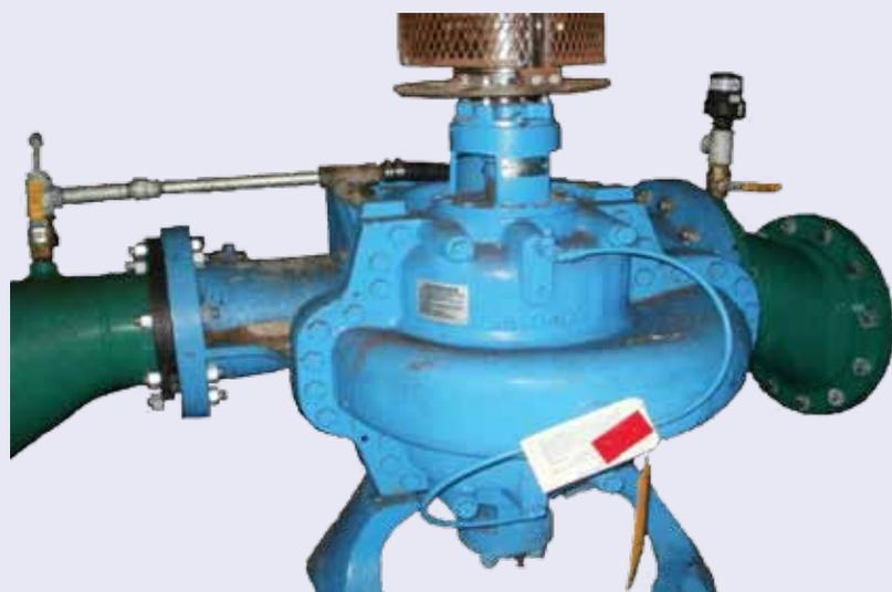
Metropolitan specially fabricated spools that also incorporated special "fusion-bonded" coatings to simplify with the installation of new pumps in this existing configuration.
