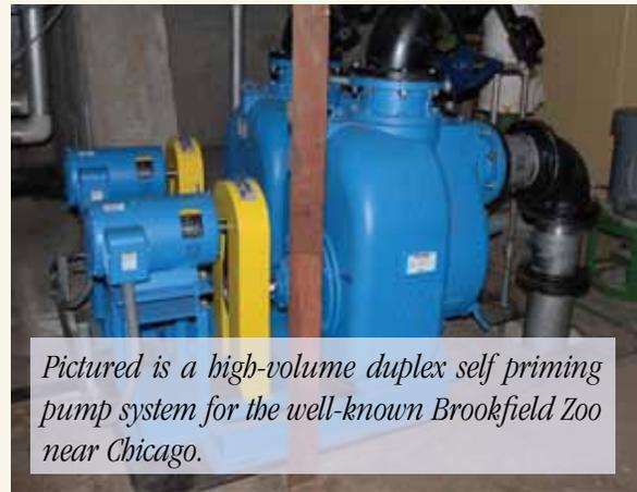
*Pictured is a high-volume duplex self priming pump system for the well-known Brookfield Zoo near Chicago.*
