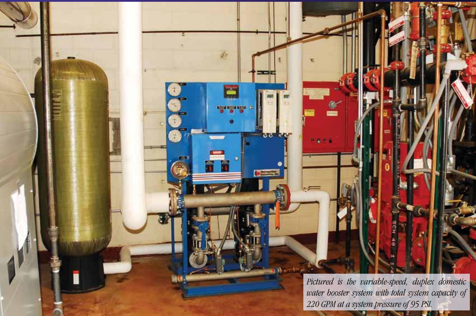
*Pictured is the variable-speed, duplex domestic water booster system with total system capacity of 220 GPM at a system pressure of 95 PSI.*
