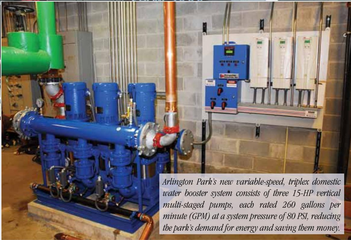
*Arlington Park's new variable-speed, triplex domestic water booster system consists of three 15-HP vertical multi-staged pumps, each rated 260 gallons per minute (GPM) at a system pressure of 80 PSI, reducing the park's demand for energy and saving them money.*
