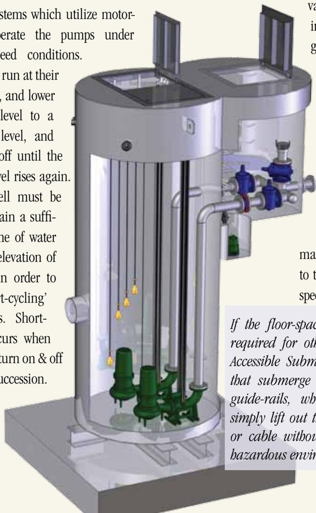
*If the floor-space above the wet-well is required for other purposes, Guide-Rail Accessible Submersible pumps are used that submerge within the wet-well; on guide-rails, which allow personnel to simply lift out the pumps using a chain or cable without the need to enter the hazardous environment of the wet-well.*
