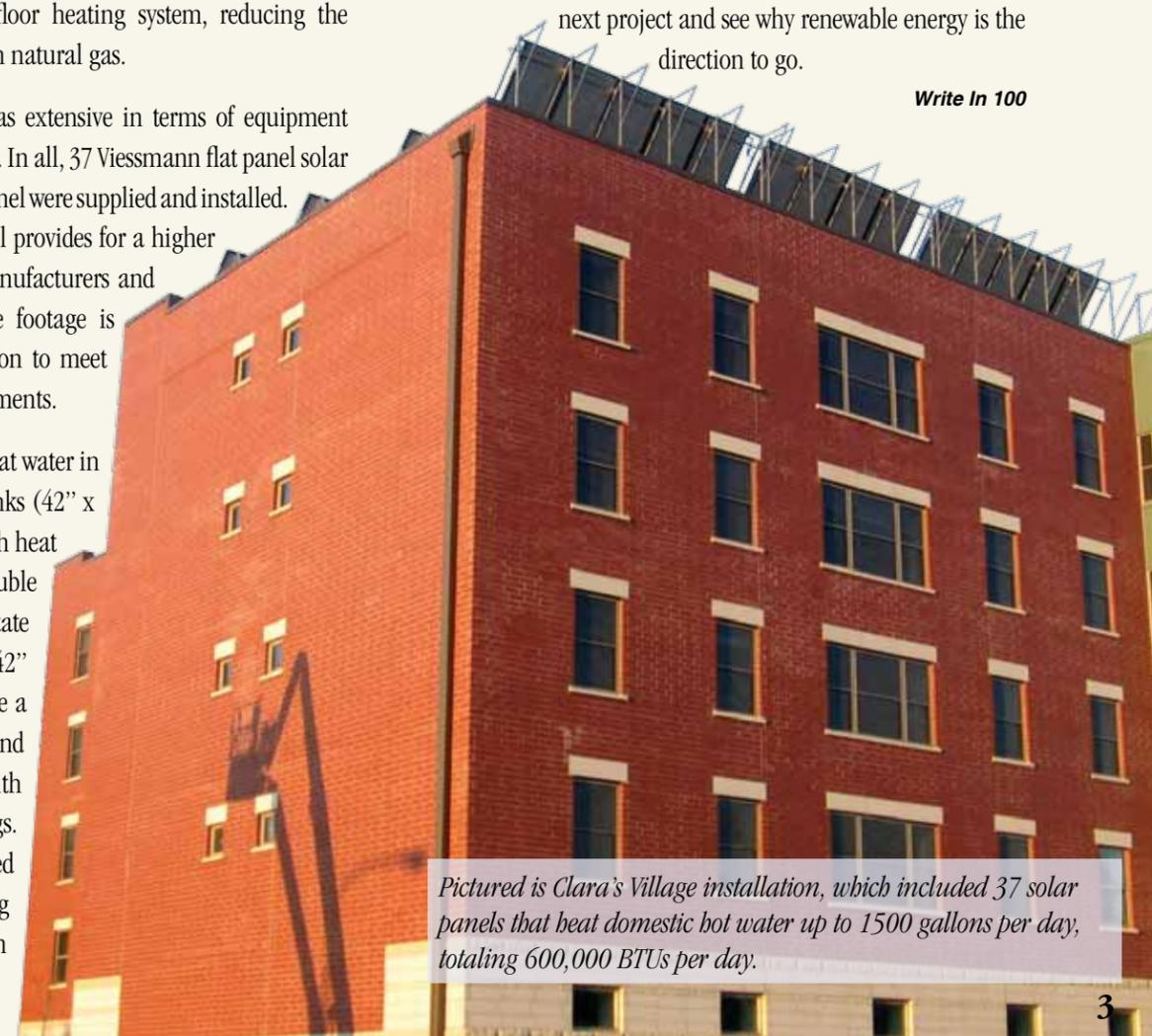
*Pictured is Clara's Village installation, which included 37 solar panels that heat domestic hot water up to 1500 gallons per day, totaling 600,000 BTUs per day.*
