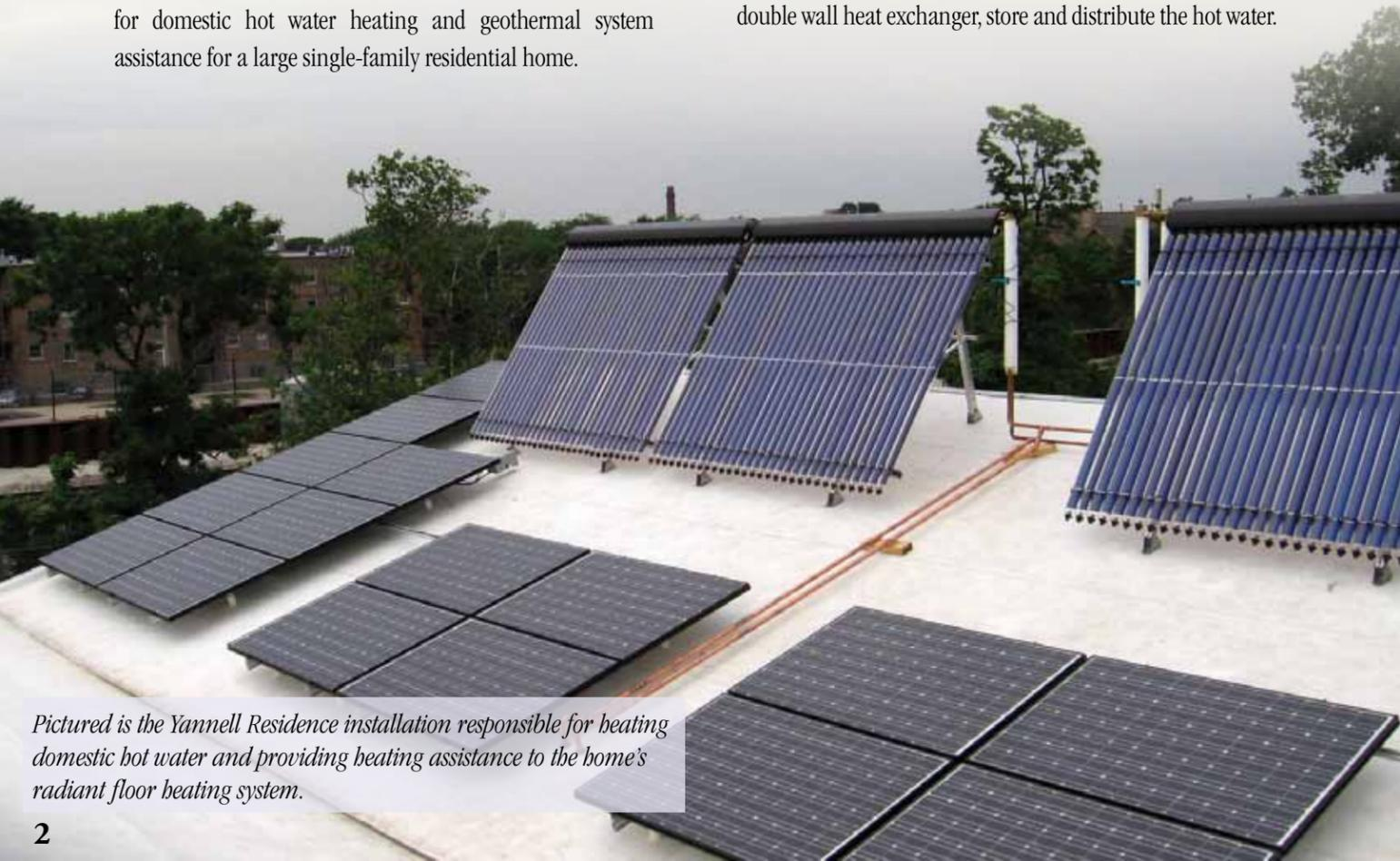
*Pictured is the Yannell Residence installation responsible for heating domestic hot water and providing heating assistance to the home's radiant floor heating system.*
