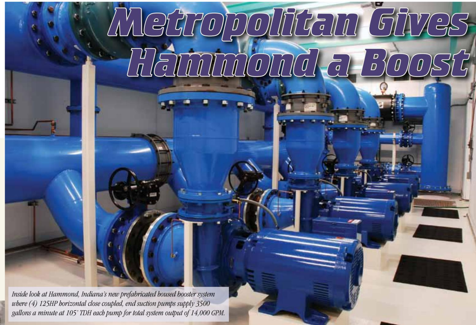
Inside look at Hammond, Indiana's new prefabricated housed booster system where (4) 125HP horizontal close coupled, end suction pumps supply 3500 gallons a minute at 105' TDH each pump for total system output of 14,000 GPM.
