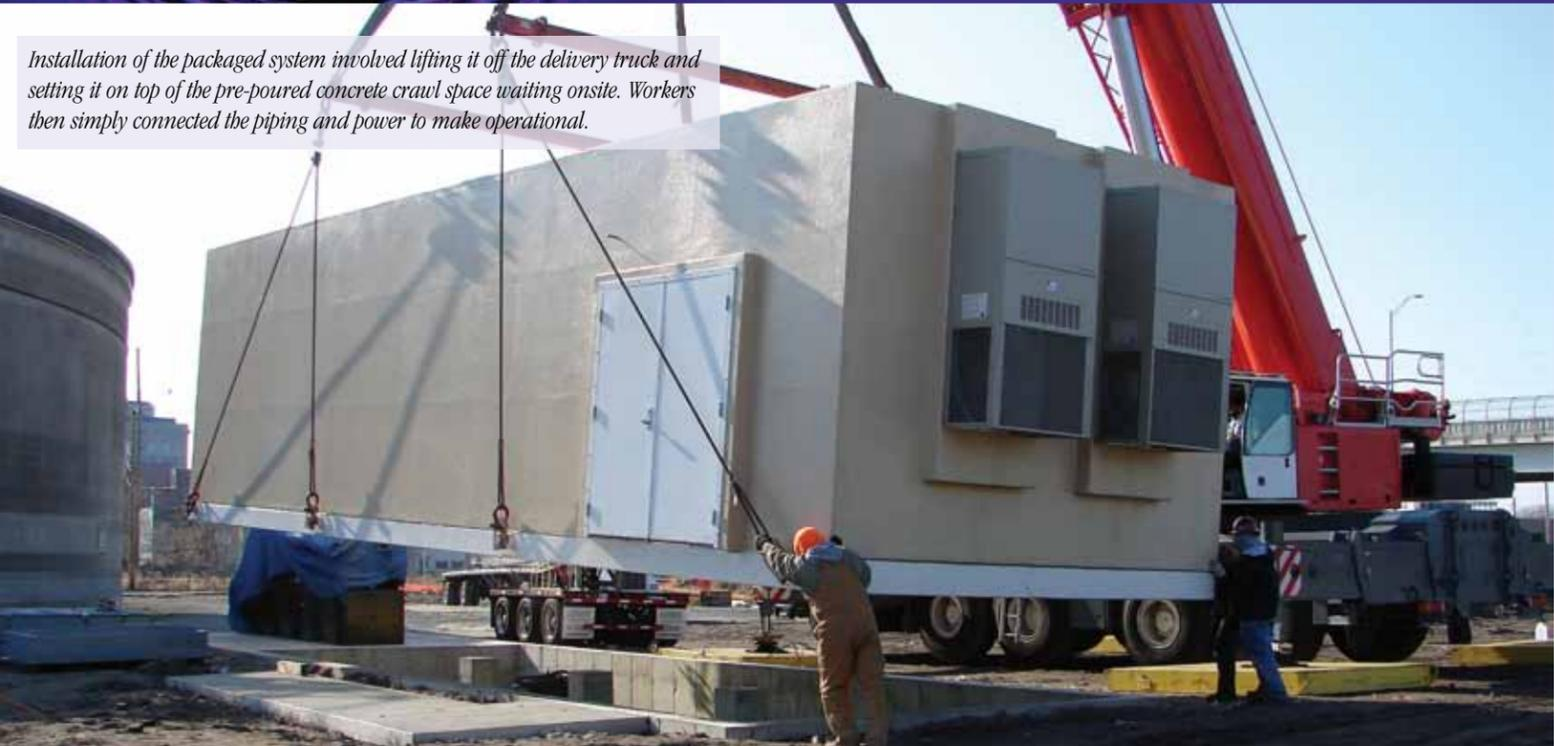
Installation of the packaged system involved lifting it off the delivery truck and setting it on top of the pre-poured concrete crawl space waiting onsite. Workers then simply connected the piping and power to make operational.
