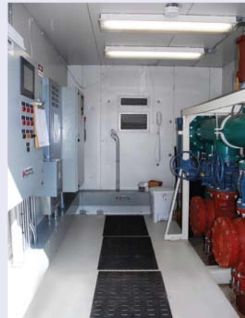
In an above grade installation, the discharge pipe and valve assembly are located inside the building for easy access.
