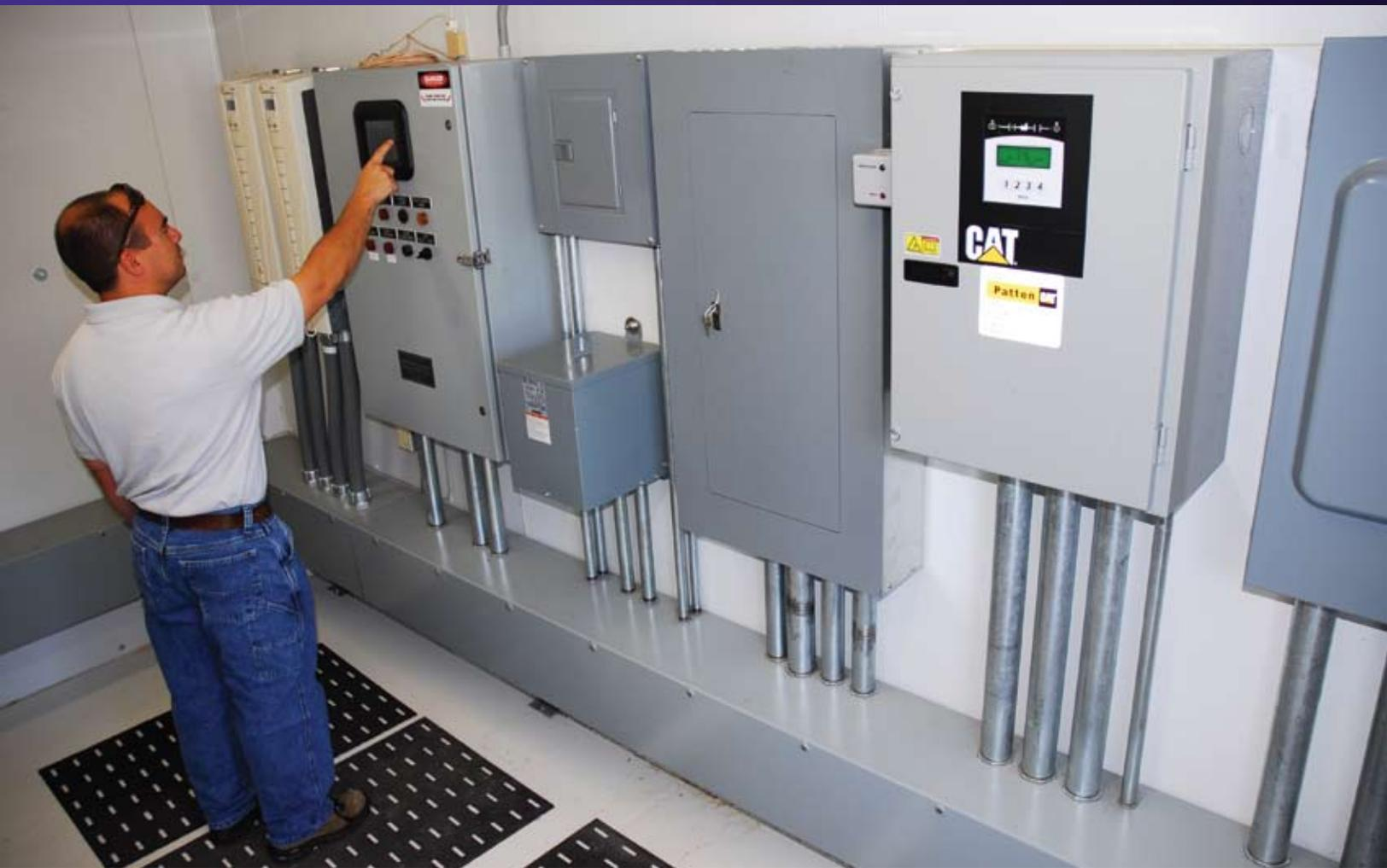
**On the control/valve side of each building, state-of-the-art controls with programmable logic controllers and touch screen operator interfaces operate the system.**
