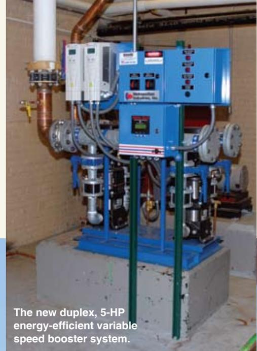
The new duplex, 5-HP energy-efficient variable speed booster system.
