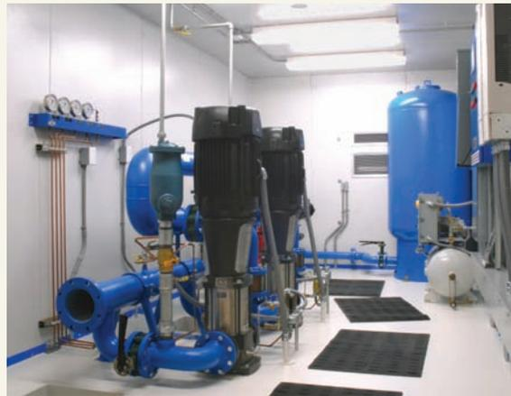
**A view inside the pump house that contains everything required for operation including pumps, motors, valves, internal piping, variable speed controls, vacuum pump, filtration system, electrical distribution equipment and HVAC equipment.**
