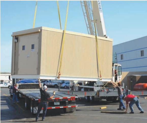
**Delivery and installation of a prefabricated housed pump station is done by simply lifting the structure and setting it on a pad. After piping in, piping out and running power, installation is complete.**
