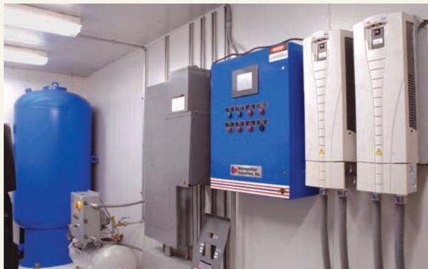
**Custom designed variable speed controls with touchscreen operate entire system, reducing equipment wear, energy and operating costs and all the while maintaining accurate pressure settings.**
