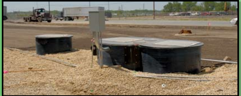
Packaged pump system for large waste transfer station using rain runoff water for truck cleaning.
