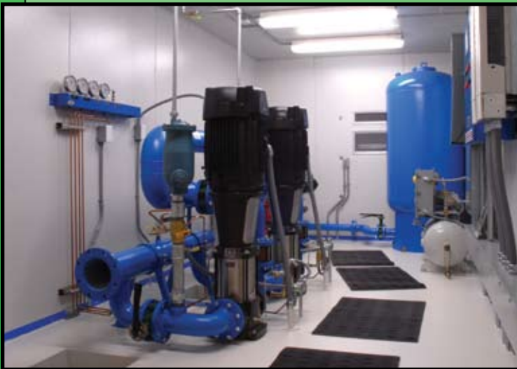
Complete packaged pump, control, and filter house which reclaims leachate for spray irrigation at a landfill.
